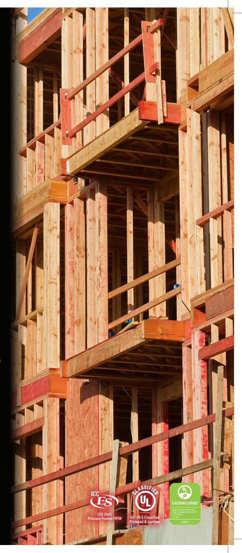
D-Blaze treated products show no evidence of significant progressive combustion after 30 minutes exposure to flame. In most applications, D-Blaze treated products offer a lower in-place cost than noncombustible-classified materials.
