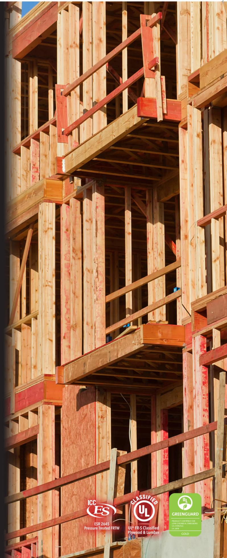
D-Blaze treated lumber and plywood is highly effective in slowing down the spread of flame and smoke development caused by fire. D-Blaze treated products show no evidence of significant progressive combustion after 30 minutes exposure to flame. In most applications, D-Blaze treated products offer a lower in-place cost than noncombustible-classified materials.
