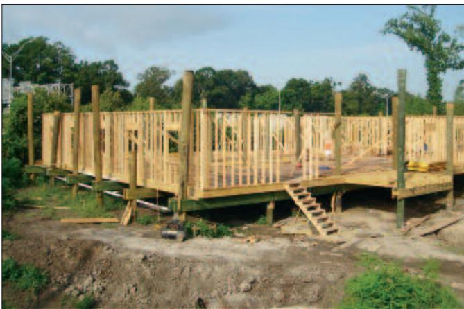
Round timber piling and glulam floor beams
