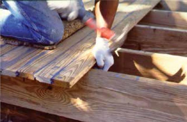
When installing the porch flooring material, begin with a coat of a mildew-resistant oil-based primer for exterior use applied to all four sides and the ends. Consider applying a coat of the final oil-based porch enamel to both the tongue and the grooves (also to the end of any piece that will be adjacent to the house) and installing it while the paint is still wet. This procedure not only assures an effective seal against moisture penetration, but also provides a good bond between floor boards.
